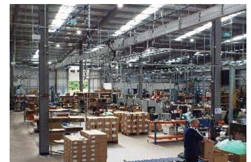
Torbay plant (UK) Completion in May 2018
