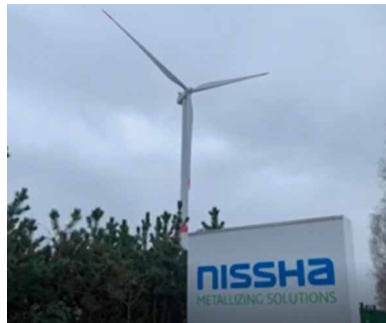
Wind power introduction: Nissha Metallizing Solutions (Belgium)
