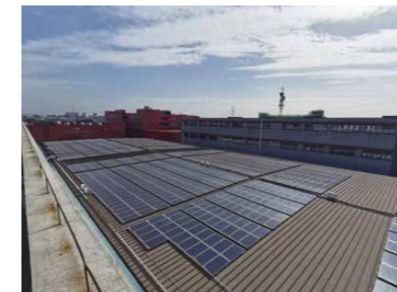
Solar power operations: Nissha (Kunshan) Precision IMD Mold (China)
