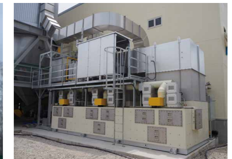
Energy-saving equipment to be introduced (thermal storage deodorizer): Nitec Industries (Japan)
